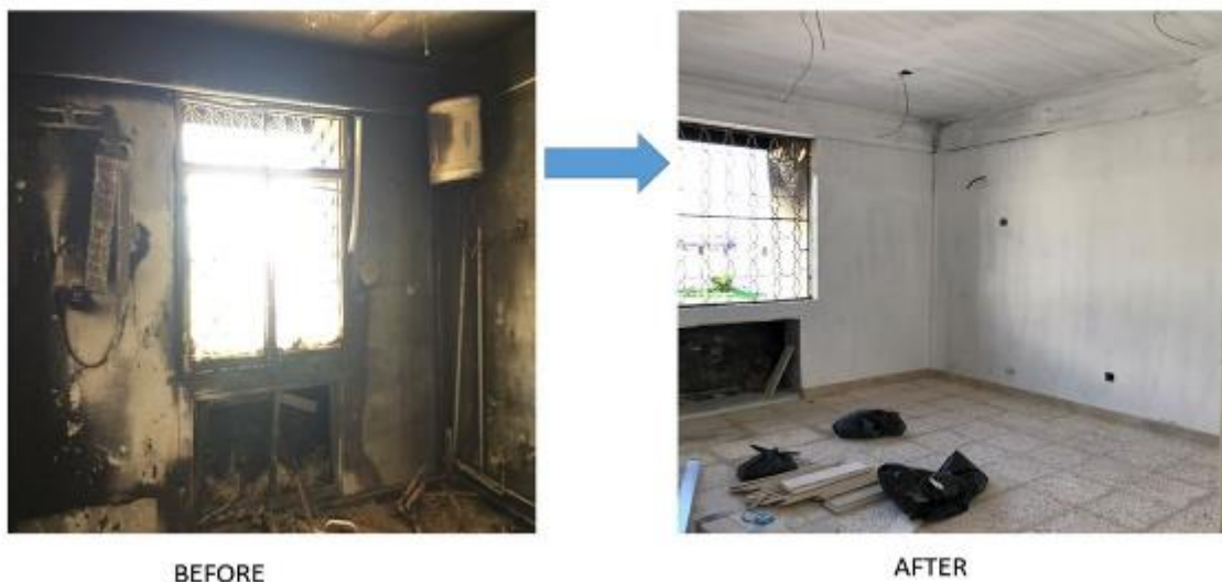
Ongoing Rehabilitation Work in the Benghazi Radio Therapy Centre
